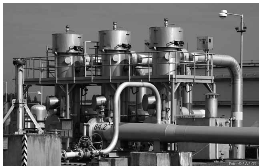
Figure 1 RWE GS underground gas storage facility
